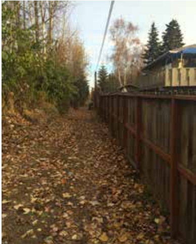
After installing new underground cable in 2014, Chugach removed its wires and cross arms from poles around the north end of Cheney Lake. Now that other attached utilities have also gone underground, a Chugach contractor will be removing the poles.
