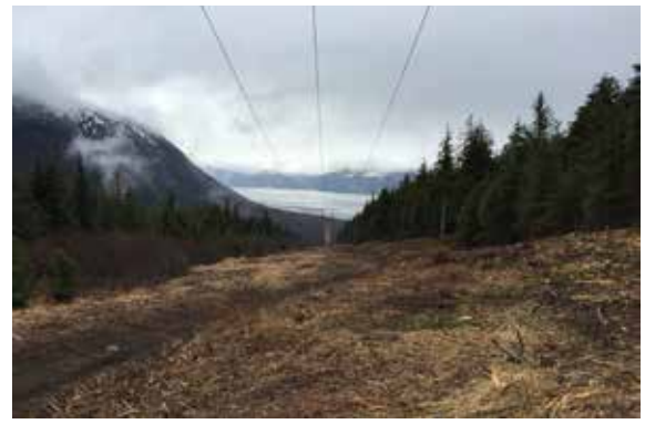
A six-mile section of the 115-kv line will be rebuilt this summer.
