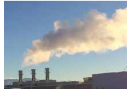
The Southcentral Power Project runs year-round, but the small amount of water vapor in its exhaust is only visible during certain winter conditions. SPP is an efficient, 200-megawatt, gas-fired power plant jointly owned by Chugach (70%) and Municipal Light & Power (30%).
