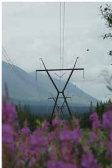
The Regulatory Commission of Alaska recently released a report examining the Railbelt transmission system
