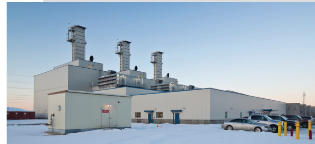
Now that the efficient new Southcentral Power Project is a utility asset, Chugach has been buying less natural gas each day.
