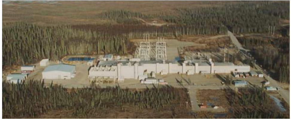
Chugach's Beluga Power Plant runs on natural gas.
