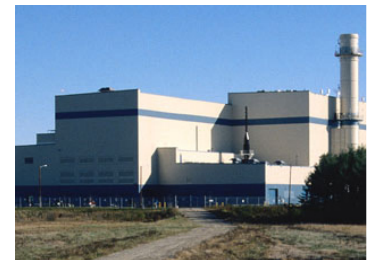
The new power plant could look similar to this one in the Lower 48
