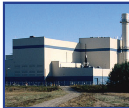
The new, efficient combined-cycle plant would be similar to the one in the photo. It would produce the same amount of power for about 75 percent of the natural gas compared to current units. The plant would consist of two gas turbine-generators and a steam turbine-generator. The term "combined cycle" refers to the fact that the hot exhaust of the combustion turbines would power the steam unit.
