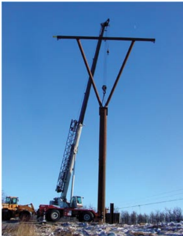
Chugach's contractor raised one of the new structures Feb. 22.
