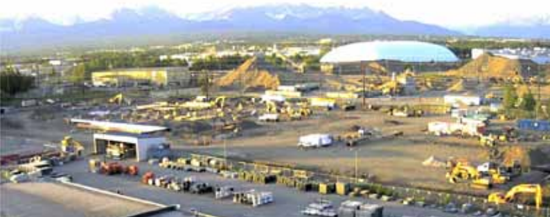
The SPP construction site in June.
