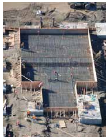
Foundations had been poured by June.
