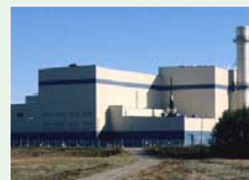
The new power plant could look similar to this one in the Lower 48
