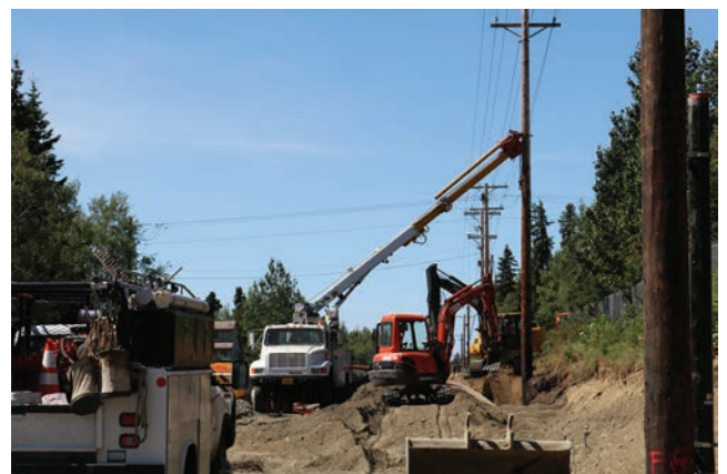
Undergrounding work in progress along Klatt Road
