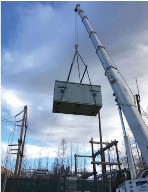
The new substation control structure lowered into the Girdwood Substation.
