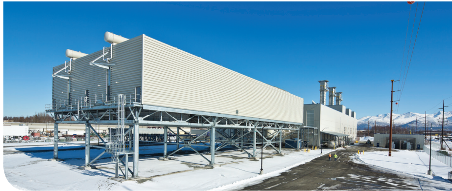
Southcentral Power Project
