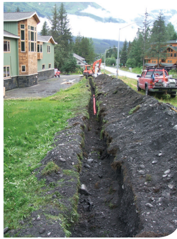
Bottom right: As part of a project to add a second feeder to serve Girdwood customers, Chugach used a state grant to install an underground feeder tie along Arlberg Road.
