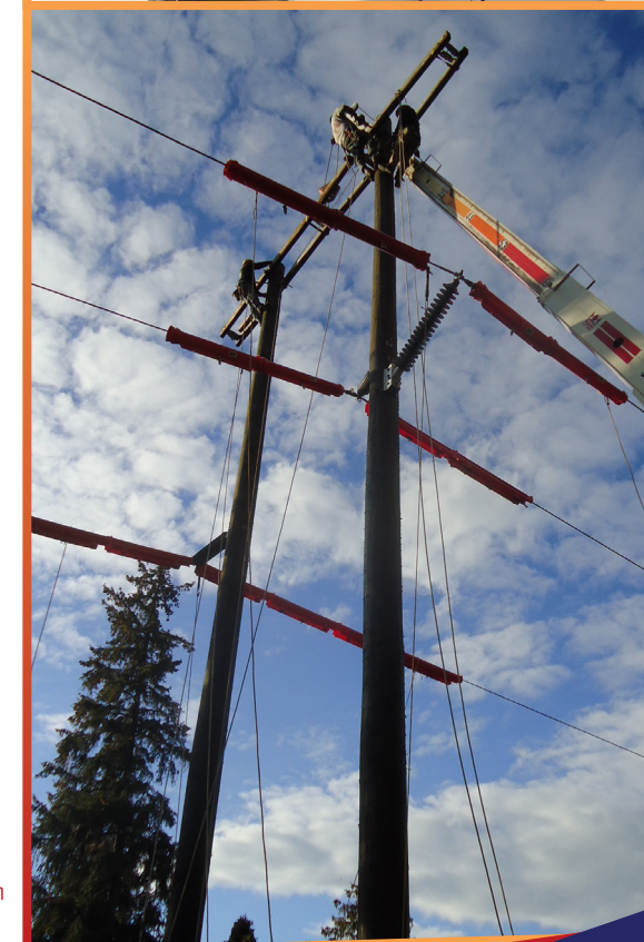
Bottom: Chugach contractor crews assembled an H-frame crossarm on the Seward transmission line repair project.
