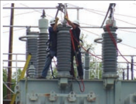
Crews performed maintenance on a transformer at the University Substation in 2008.
