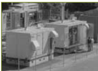
On Aug. 9 Chugach added a 1-Mw fuel cell to its grid. The project provides assured power for a Postal Service Center, as well as power for other customers on the grid.
